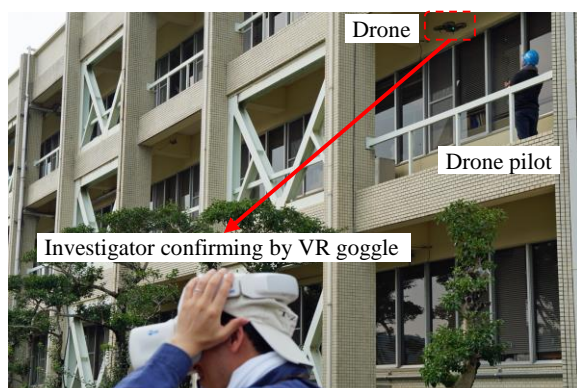
Figure 15. Remote investigation by drone in damaged building.
