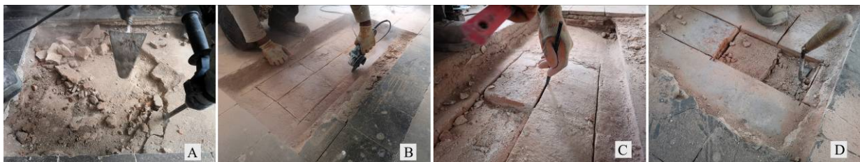
Figure 5: The sequence of operations of the extractions of samples from the timbered vaults: (A) removing the pavements and the vault filling, (B) removing the mortar between tiles by using a radial saw, (C) extracting the tiles with a chisel, (D) extracting the tiles with a gauging trowel.
