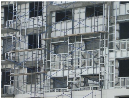
Fig. 3. The protecting constructions of the high-rise building with filling a foamconcrete into the fixed formwork.
