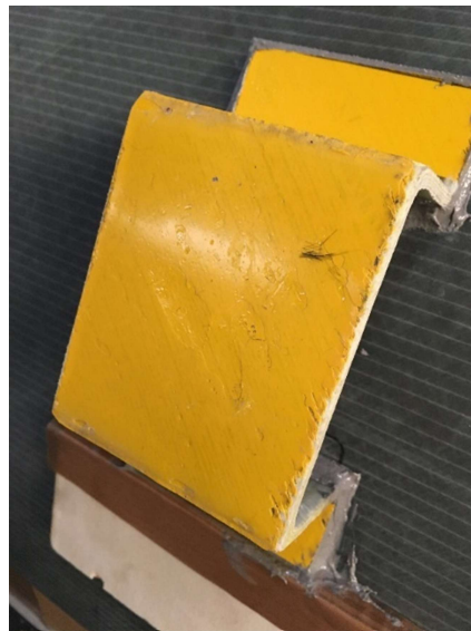
Figure 33 : cable tray support with dry coating
