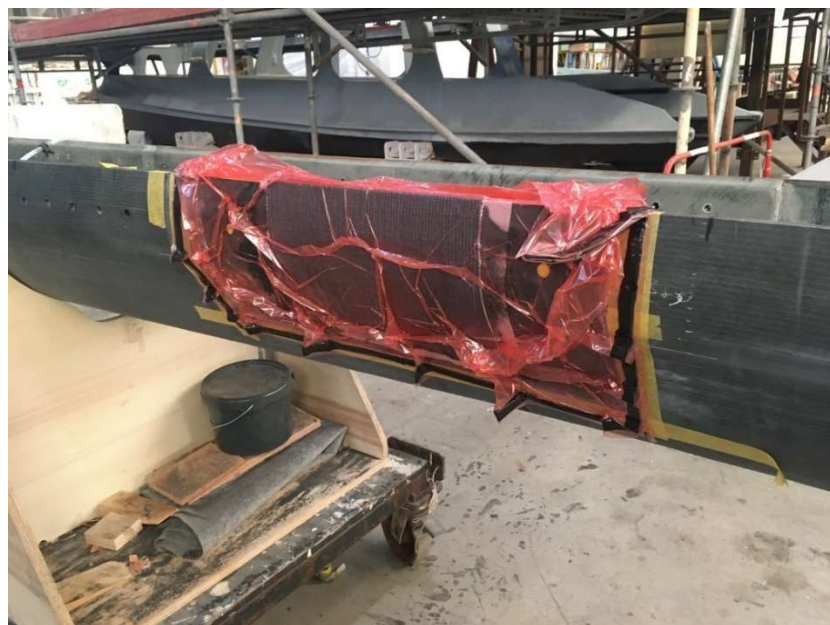
Figure 28 : Repair under vacuum
