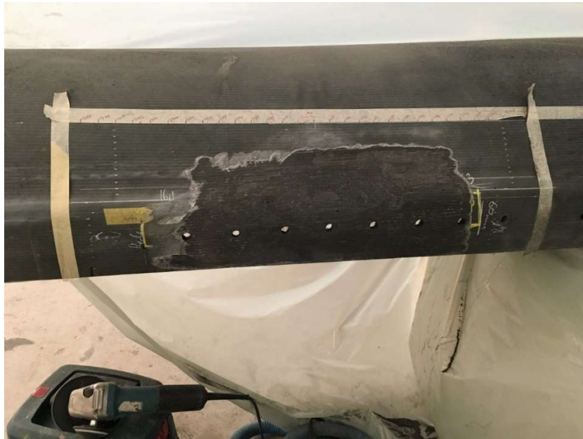
Figure 27 : grinding of the area
