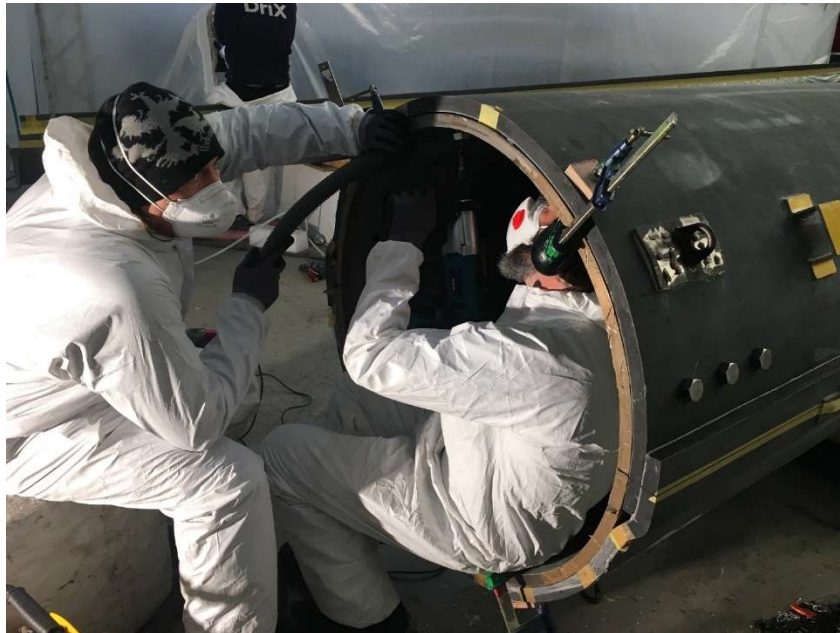
Figure 29 : drilling for bottom ring assembly
