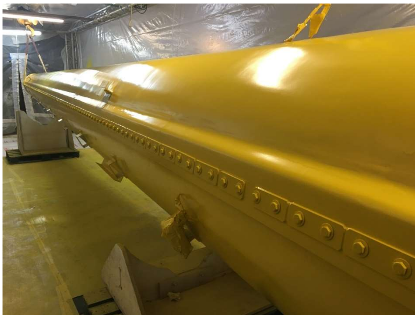
Figure 40 : Mast with topcoat
