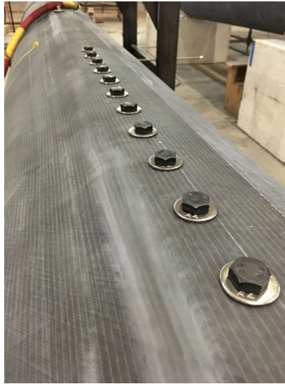
Figure 25 : Temporary bolting
