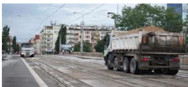
Figure 3: Vehicles during static load test – crossing
