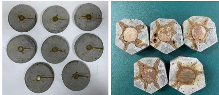
Figure 10. Crack pattern in the smooth-R/ECC (left) and ribbed-R/ECC (right).
