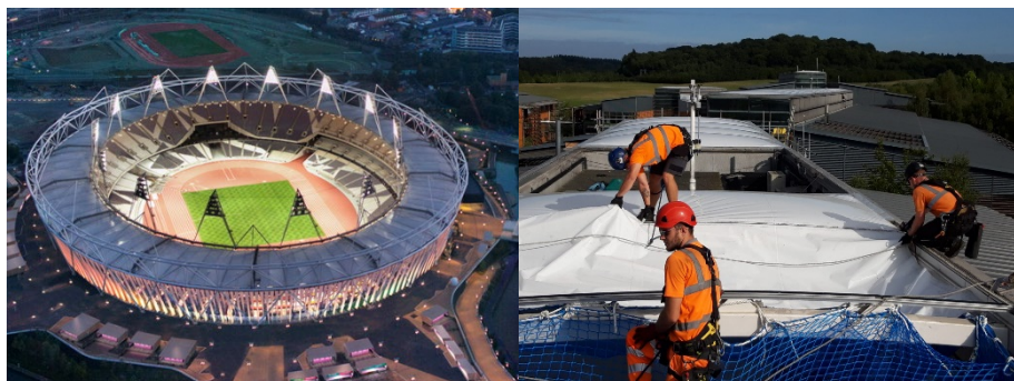
Fig. 2. Left: London Olympic Stadium, 2012© Populous, right: Dismantling ETFE foils, Vodafone project © Vector Foiltec
