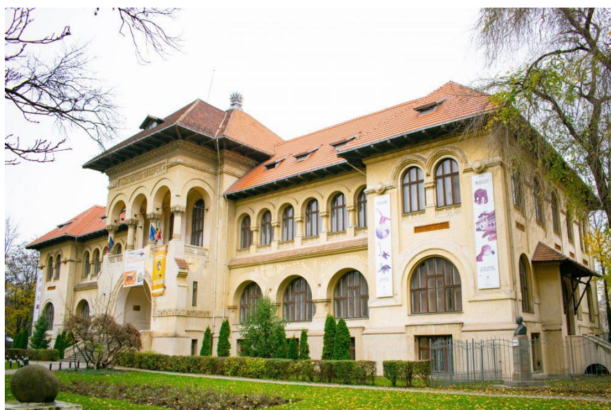
Figure 3: Main facade of the National Geological Museum
