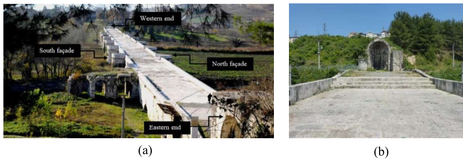
Figure 2: Justinian's Bridge; (a) view of the bridge today [14], (b) apse structure [16].
