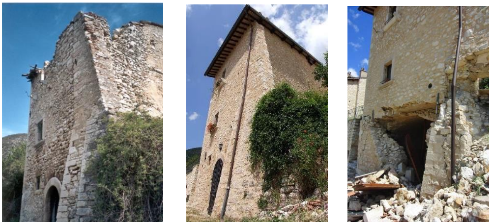
Figure 4: Photos of the case study: a) after 1997 earthquake b) after the restoration in 2000s c) after the earthquake in 2016.
