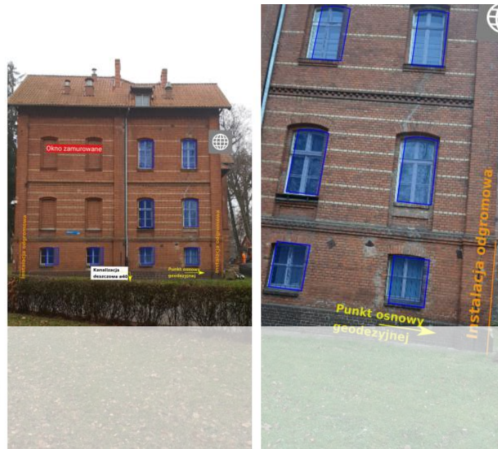
Figure 3. Additional, sample information about building facade presented in AR mobile application.
