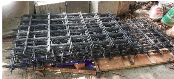
Figure 2. 8 mm Weled Wire Reinforcement (WWR)
