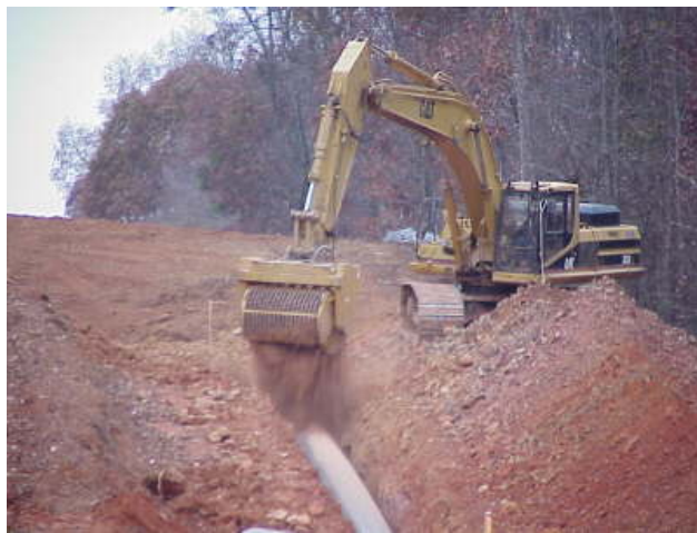
FIGURE 3.3-14 Backfilling Pipeline (Source: Photos courtesy of U.S. Pipeline, Inc. Reproduced with permission.)
