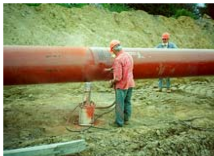
FIGURE 3.3-12 Applying Coating to Pipeline
