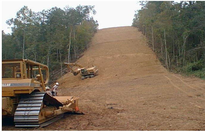
FIGURE 3.3-15 Final Contouring of Pipeline ROW (Source: Photo courtesy of FERC)
