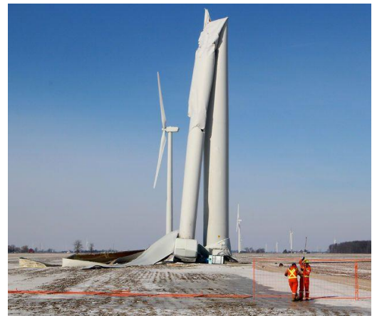
Figure 242 – Buckling failure of a wind tower [91]
