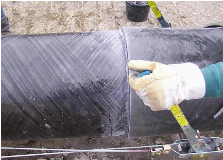
Figure 64 – Adhesively bonded pipework for offshore application
