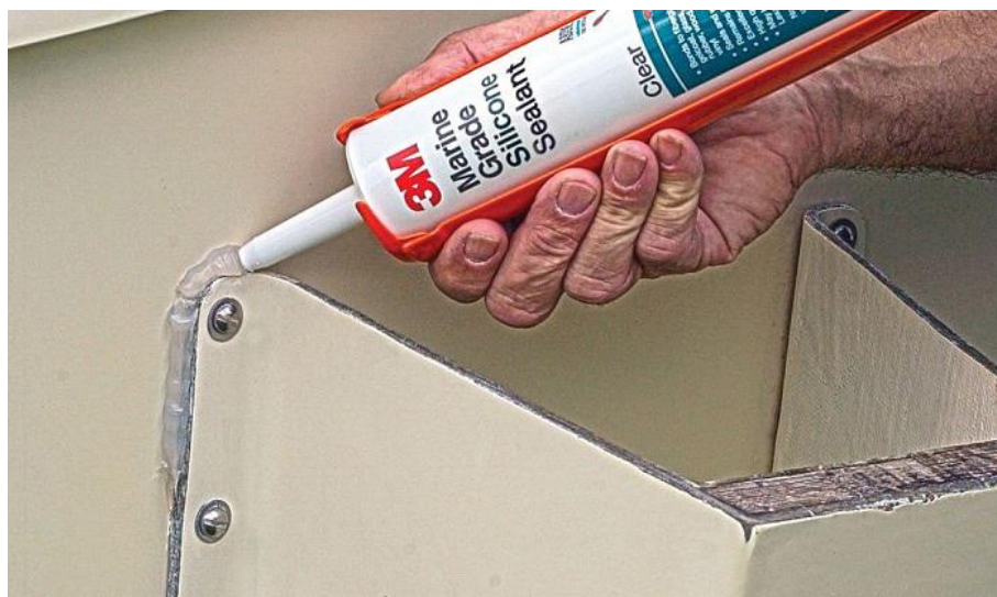
Figure 66 – Example of application of a silicone sealant in a marine structure
