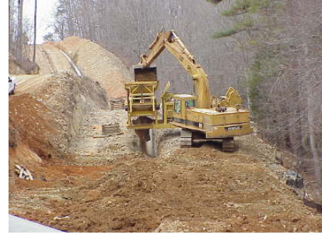
FIGURE 4.1-2 Pipeline Trenching Operations (Source: Photo courtesy of U.S. Pipeline, Inc. Reproduced with permission.)
