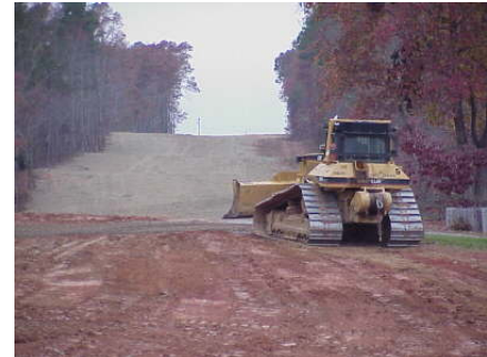
FIGURE 4.1-1 Bulldozer Grading Pipeline ROW (Source: Photo courtesy of U.S. Pipeline, Inc. Reproduced with permission.)
