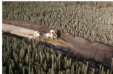
FIGURE 4.1-7 Trench Backfilling Operations (Source: TAPS 2007)
