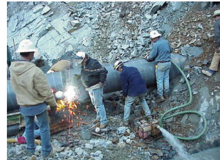
FIGURE 4.1-4 Pipeline Welding (Source: Photo courtesy of U.S. Pipeline, Inc. Reproduced with permission.)
