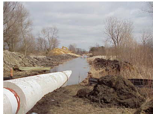
FIGURE 4.1-13 Pipeline for Wetland Installation Encased in Concrete to Counteract Positive Buoyancy (Source: Photo courtesy of U.S. Pipeline, Inc. Reproduced with permission.)
