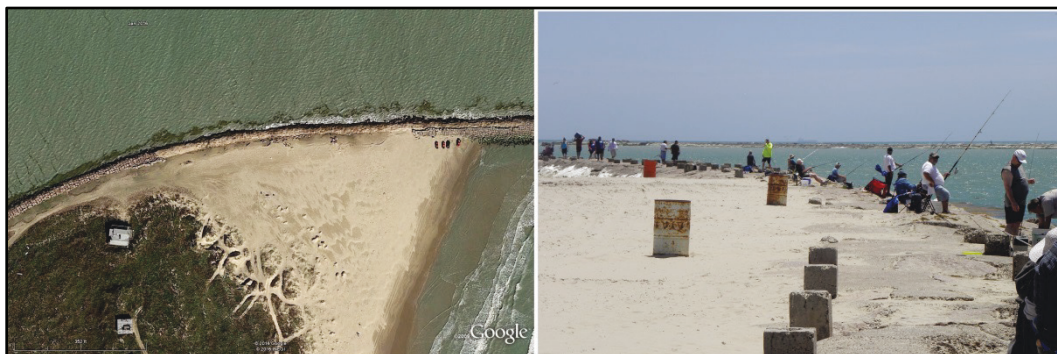
Figure 8-14. Brazos Santiago Inlet south (left panel) and north (right panel) jetties at dune line showing sand level near the crests of the jetties.
