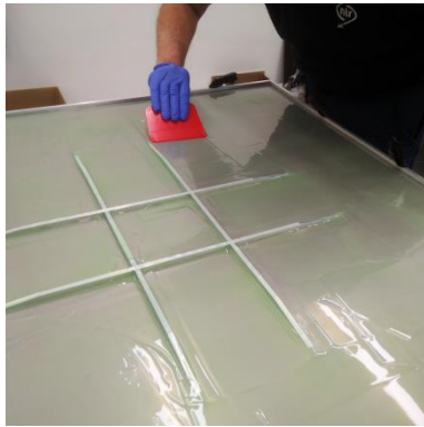
Figure 10: Silicone being applied to aluminium plug
