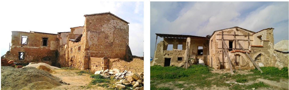
Figure 2: Photographs of the east part of the Potamia Manor showing stone masonry structures facing towards the north (left) and adobe constructions attached to stone structures at the south (right).
