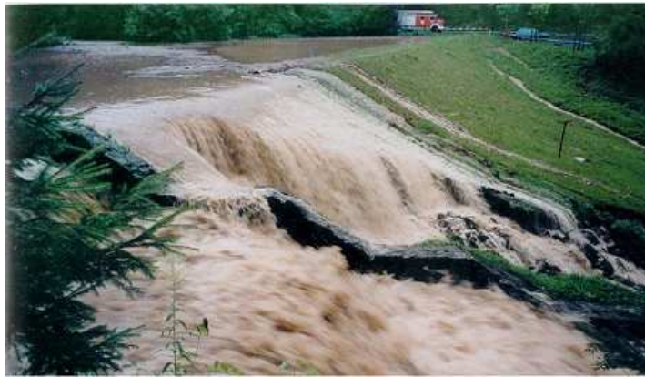
Figure 1.3: Glashütte embankment dam (Germany). Image taken from [30].
