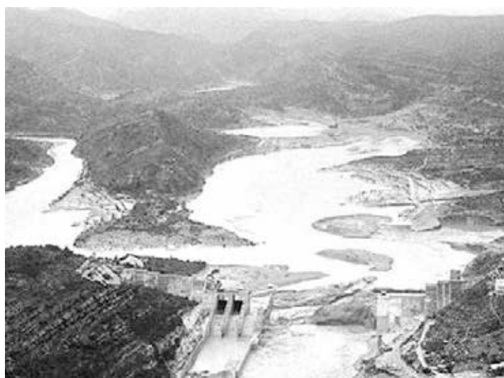
Figure 1.2: Image of Tous dam after the overtopping of October 19th, 1982.
