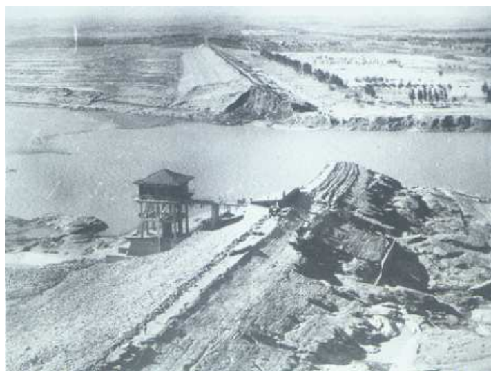
Figure 1.1: Image of Banqiao dam. Image taken from [1].
