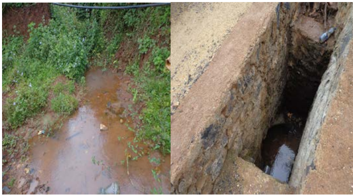
Figure 3.2. Ground water as observed on the surface.
