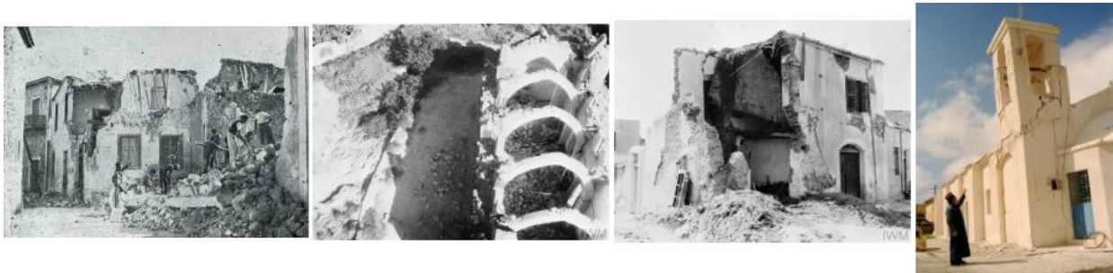
Figure 4: Structures in Cyprus damaged by earthquakes [18]
