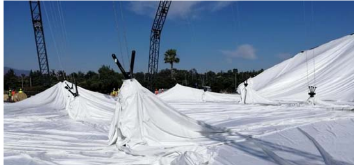
Figure 21: lifting of the main membrane
