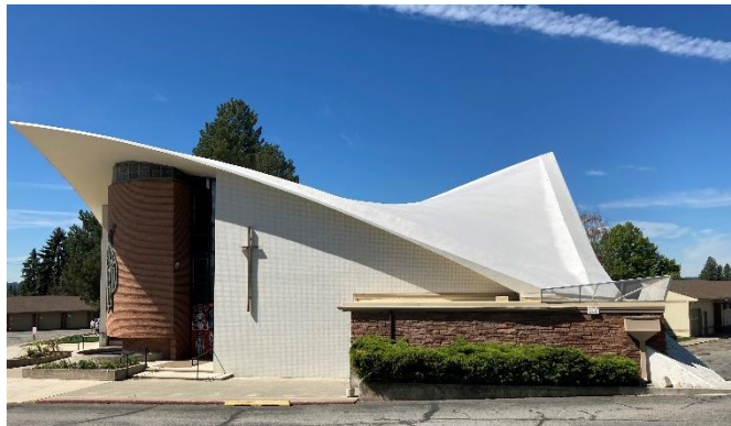
Figure 1: Hypar Roof at St Chales, Spokane, WA in 2022.
