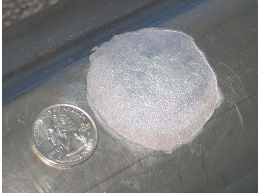
Figure 5.12: Top view of accelerated corrosion, 10% through thickness
