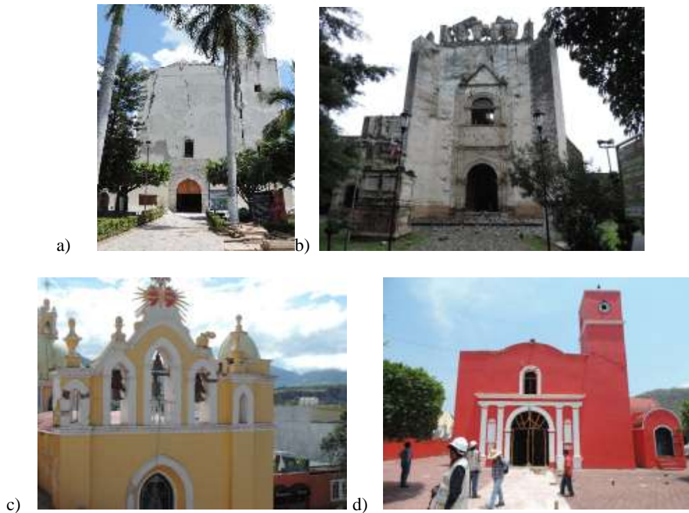
Figure 2: Damages patterns in façades: a) Tlaquiltenango, Morelos; b) Tlayacapan, Morelos; c) Huajuapán de León, Oaxaca and d) Chila de la Sal, Puebla
