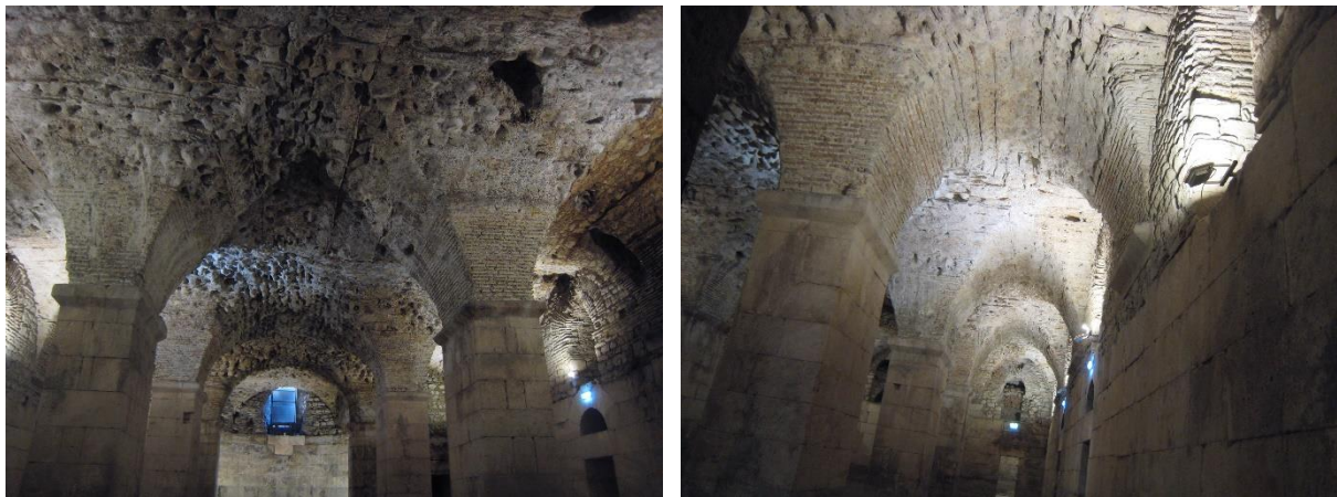
Figure 3: The largest hall in the western part of the substructures: cross vault in the central aisle (left) and in the side aisle (right) (photograph by the author)
