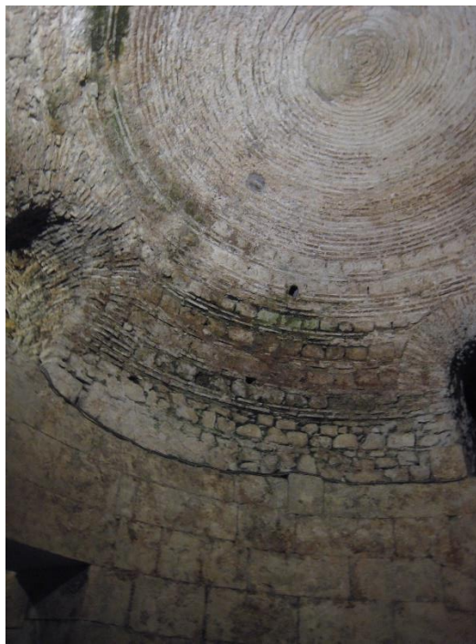
Figure 5: Dome of the circular room (photograph by the author)
