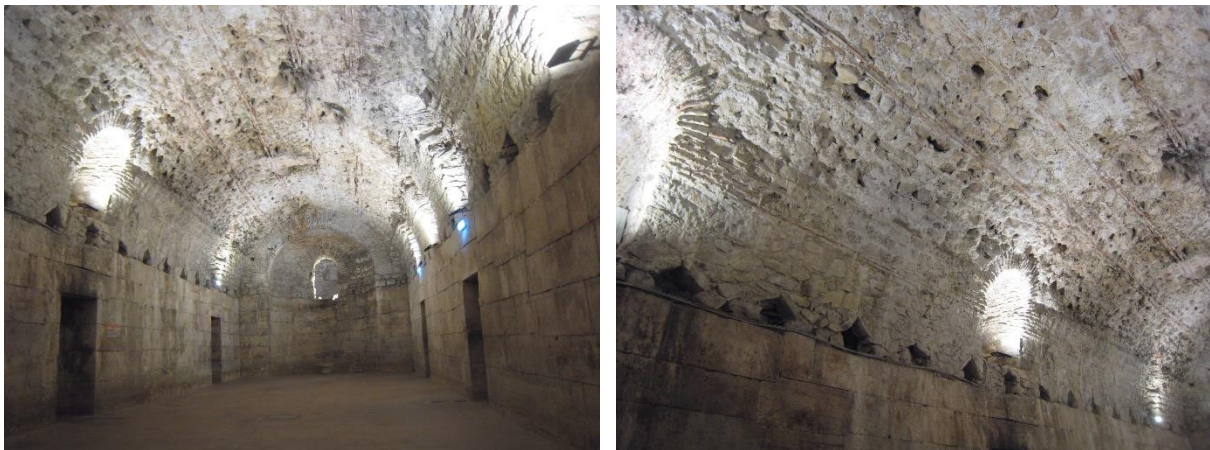
Figure 4: Barrel vault of the smaller longitudinal hall of the substructures (photograph by the author)
