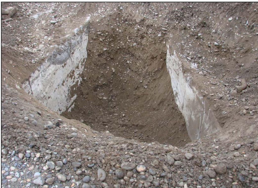
Figure 12. Intake and Exhaust Ducts to the 119-F Stack Filter Building During the 100-F-46 Excavation.
