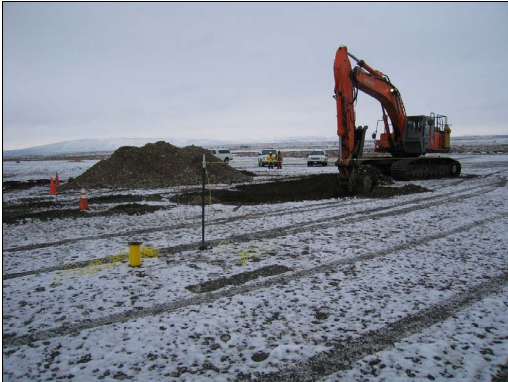
Figure 10. Excavation of the 100-F-46 Waste Site.
