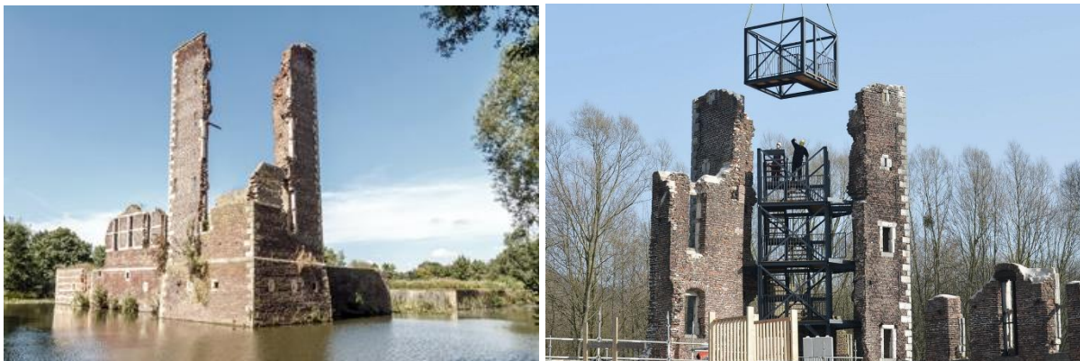
Figure 2: The remaining tower of Schaesberg castle before (left) and after (right) the latest consolidation.
