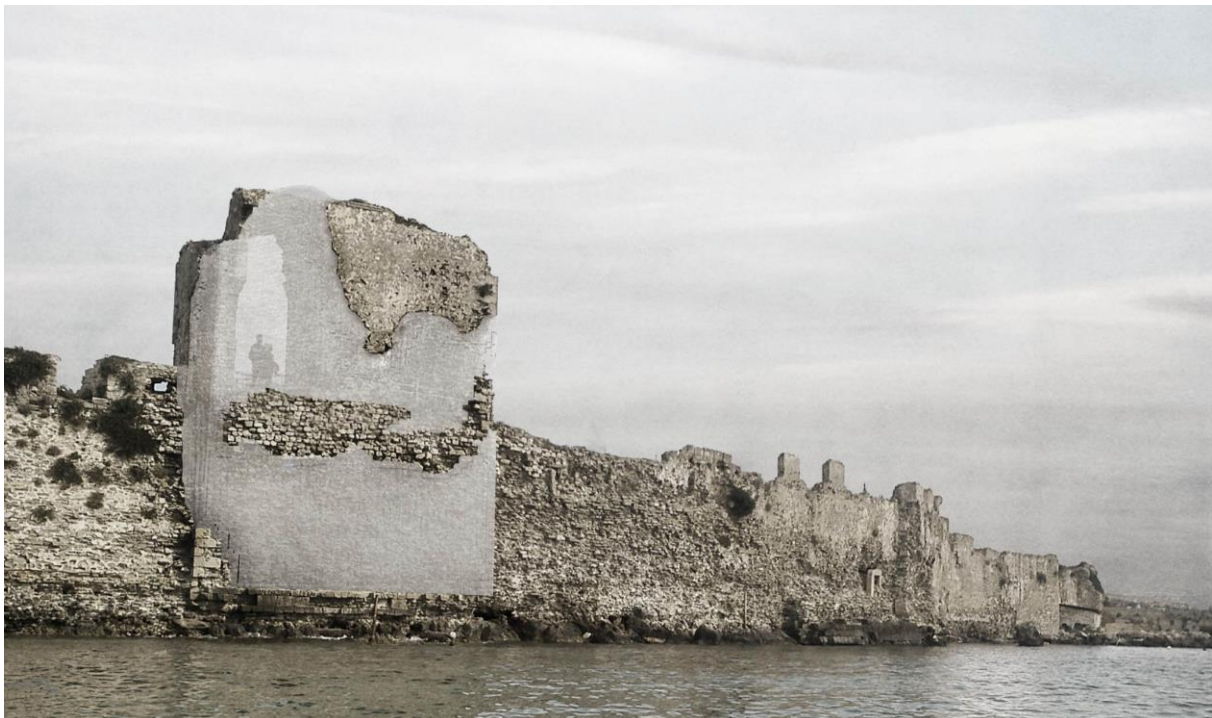
Figure 1: Fill-in-Glass Restoration design proposal for the consolidation of Bembo's bastion in Greece [6].
