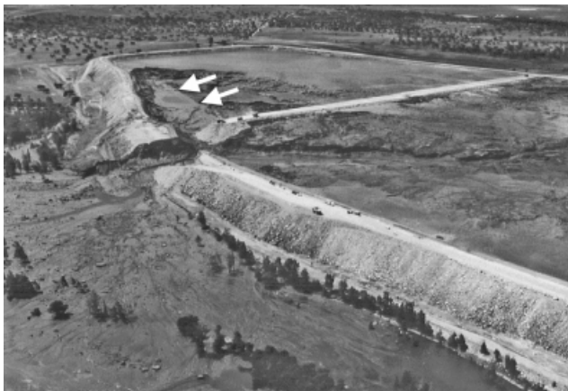
Fig. 19. The straight line, indicated by arrows, shows the position of the upstream scar of the slide
