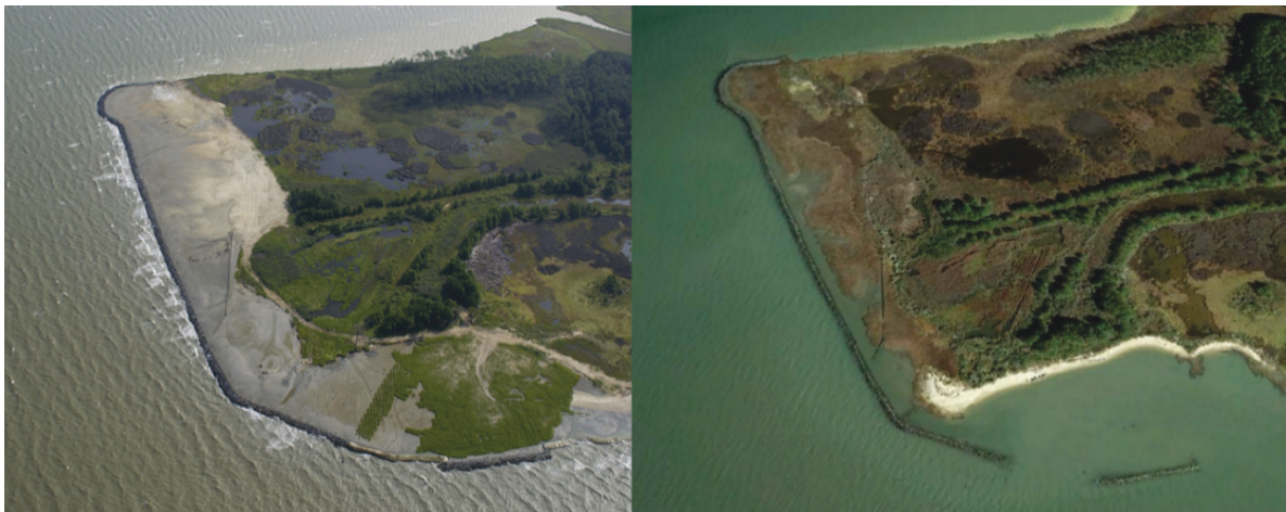
Figure 5. Barren Island north shore restoration before (left) and after (right) wetland plantings.
