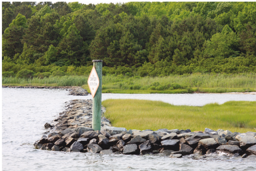
Figure 3. The opening created in the Isle of Wight breakwater allowing for natural tidal flows within the marsh.
