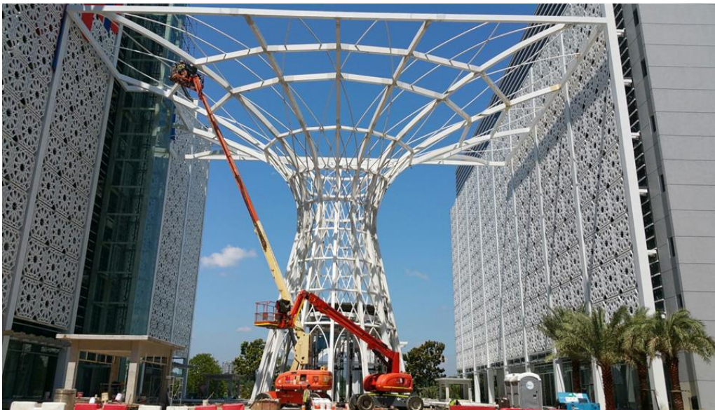
Figure 13: Completion of the supporting single layer space frame
