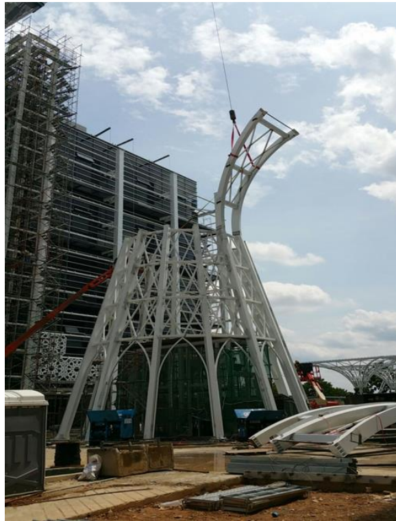
Figure 12: Construction of supporting single layer space frame
