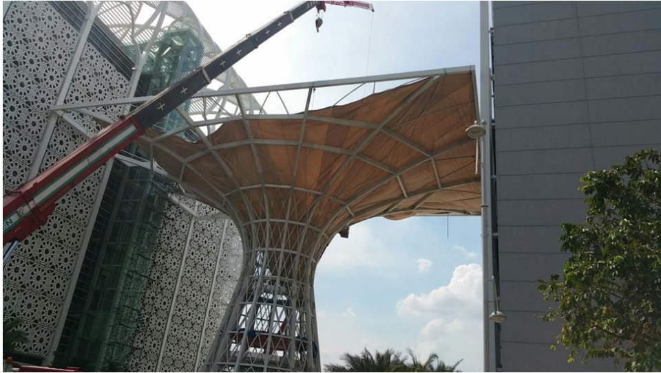
Figure 14: Installation of the PTFE membrane
