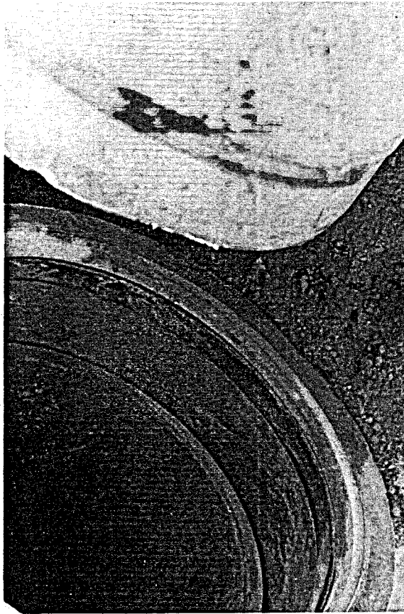
Fig. 2 View of coupling gasket between pipe sections
