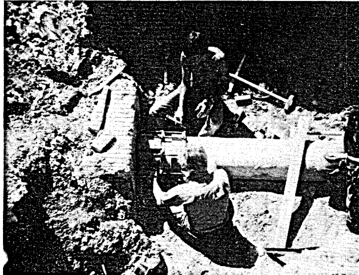
Fig. 5 Blocking Dresser coupling so that thermal cycling could not cause it to move and leak.
