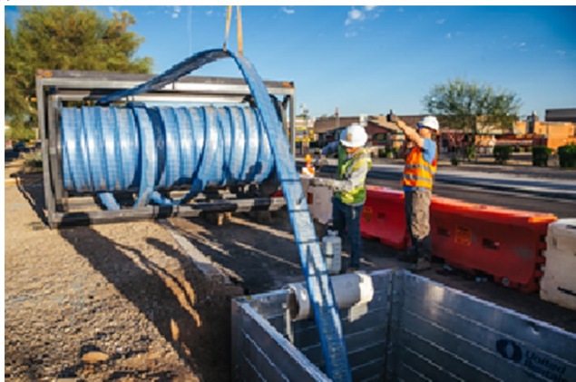
Fig. 3. Flexible hose on the reversing drum.
