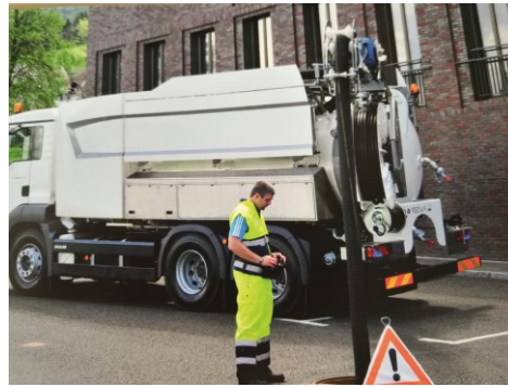
Fig. 1. Pipeline cleaning and inspection.
