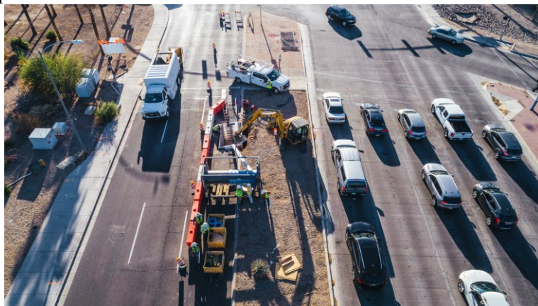
Fig. 4. Pipeline rehabilitation on the public roads.
