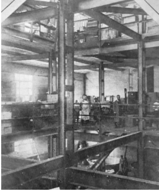
Figure 11: Interior of La Estrella soap factory (Source: German progress in America, 1924).
