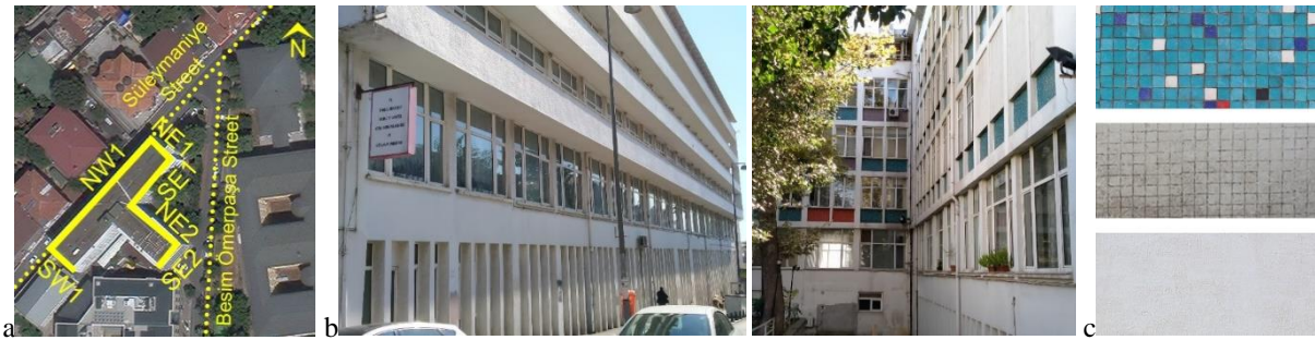
Figure 1: a) Close surrounding (straight lines represent examined façades and they have numbered according to its orientation and repetition) (URL-3), b) Views of the façade (Authors, n.d.); NW1, SE1 and NE2, c) Façade finishing materials (Authors, n.d.); colorful mosaic ceramic, mosaic ceramic-painted, and rendered-painted.
