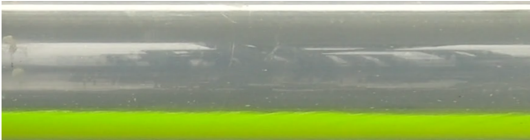
Figure 5 - Example of a cropped image from the pipe section between markers.
