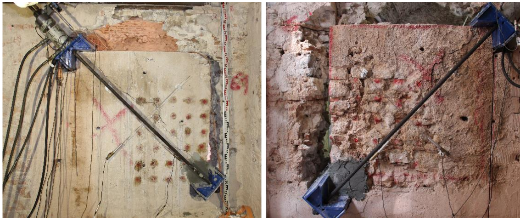
Figure 2: Cracking paths on CD01 specimens after the DC test, side 1 and 2.
