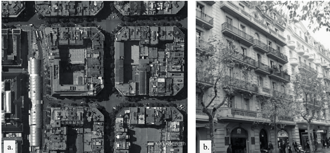
Fig. 2 Analyzed building located in Barcelona. a) Aggregate; b) Façade
