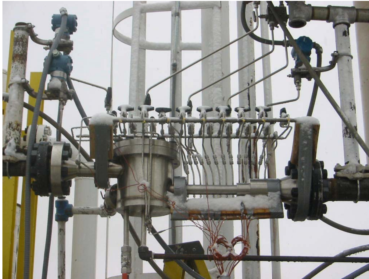
Figure 47 Single Nozzle Test Installed at CEESI
