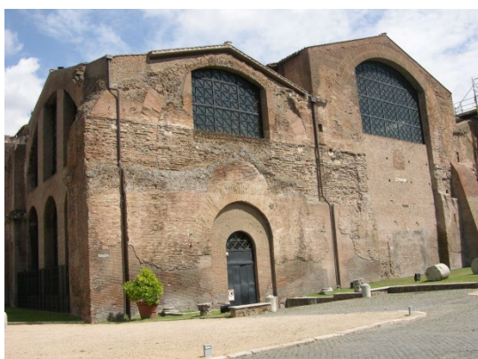
Figure 1: Side photograph of Hall I
