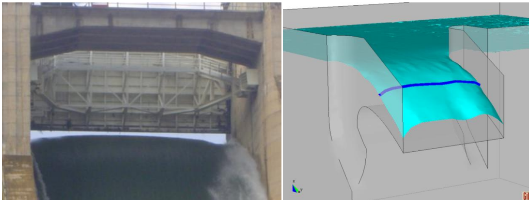
Figure 10. Shape of the free surface for free flow. Left: Actual Oliana Dam spillway. Right: Numerical model
