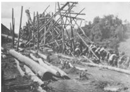
Figure 8. People of Dayak erected a pillar ( jih ) of Betang (Source: Tropen museum, the Netherlands.)
