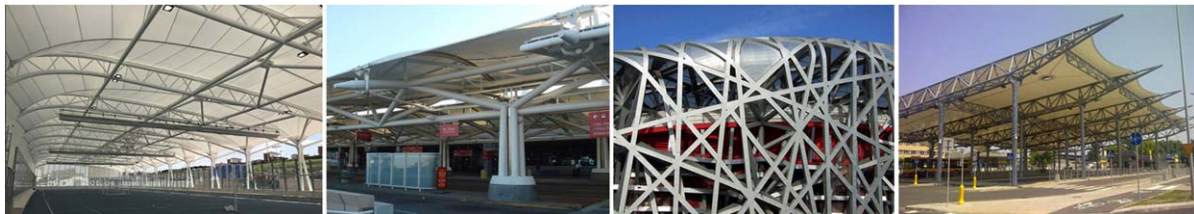
Membrane structures frequently end up being conventional steel structures.
