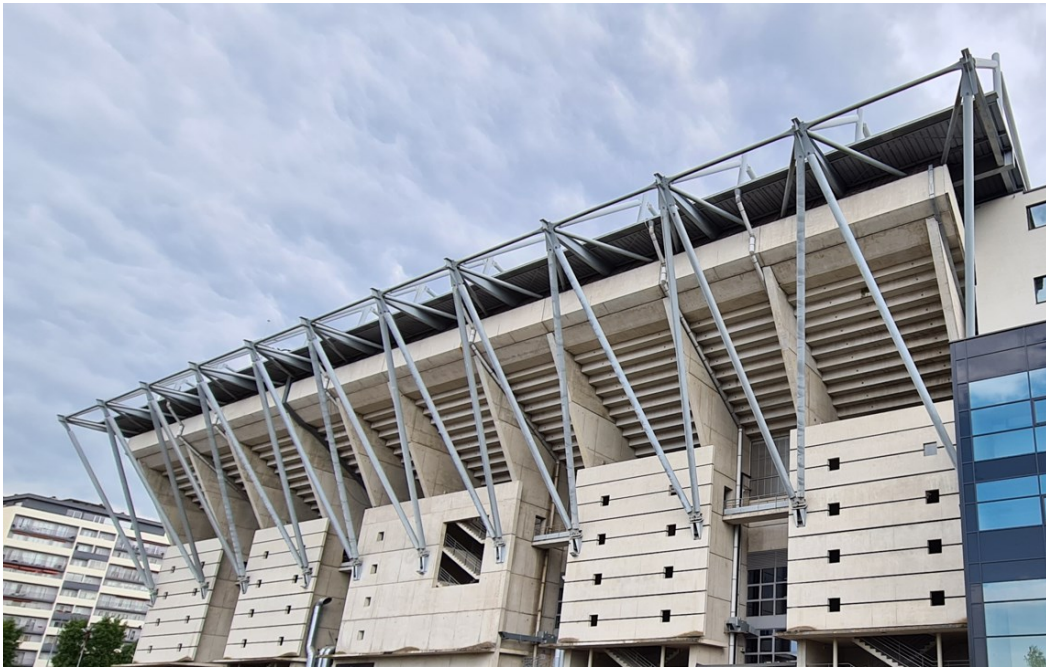
Figure 2: Membrane covering is proposed on west side existing steel structure (source: formTL)
