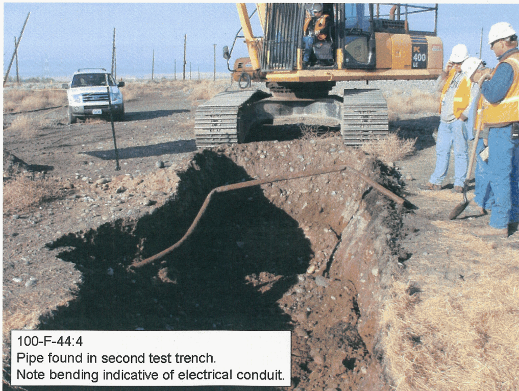
Figure 5. 100-F-44:4 Site With Pipe in Second Test Trench.
