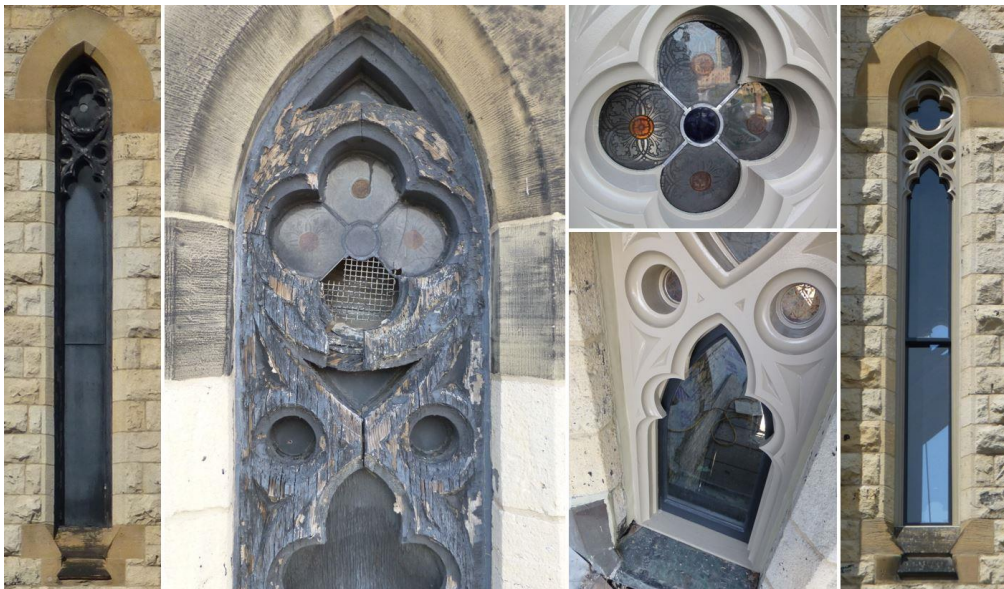
Figure 1. Typical window conditions before (left) and after restoration (right).
