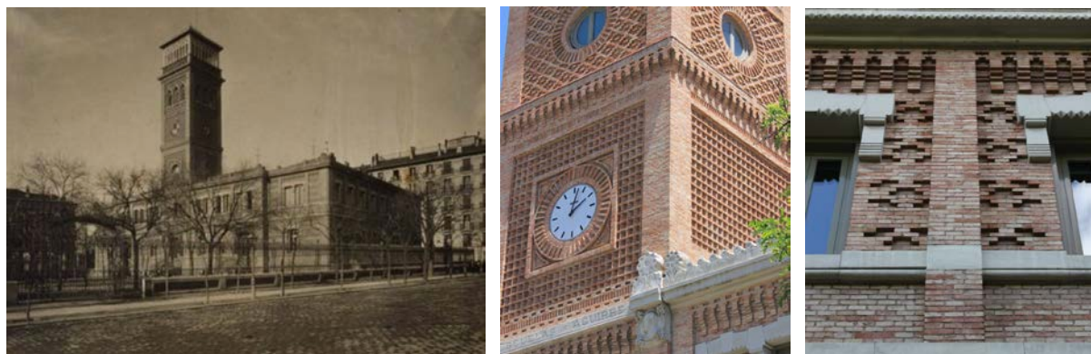
Figure 1a. The Escuelas Aguirre building in the 1920s. (Lacoste, circa 1925). Figures 1b and 1c. Some views of the brick bonds in different areas of the façade. [1]
