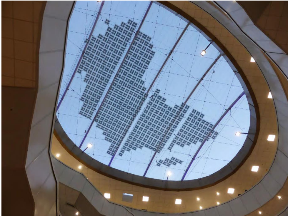
Figure 9: ETFE cushion atrium roof including photovoltaic modules
