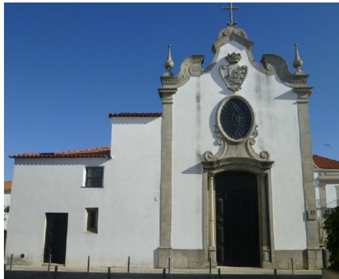
Figure 2: Main façade of the church.
