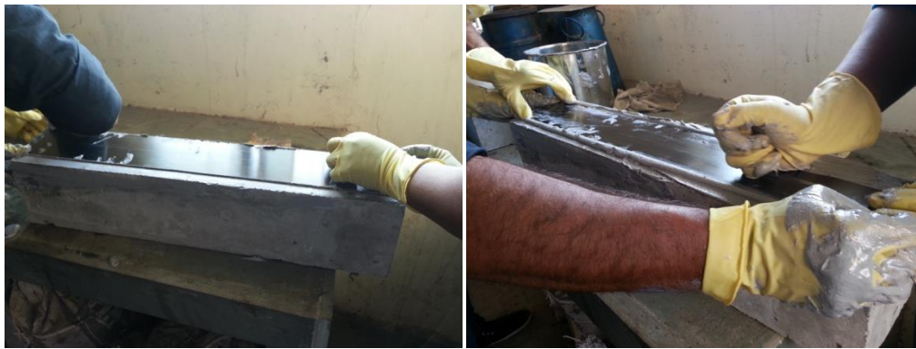
Fig. 6: Install the laminates on beam
