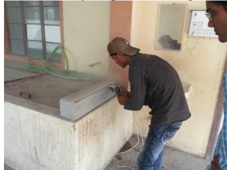
Fig. 1: Grind the surface
