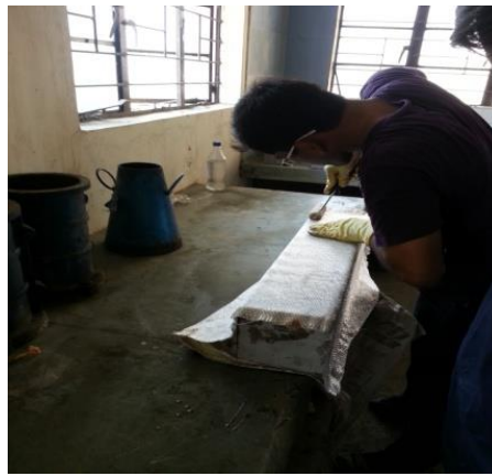
Fig. 4: Applied glass fibre wrap on beam
