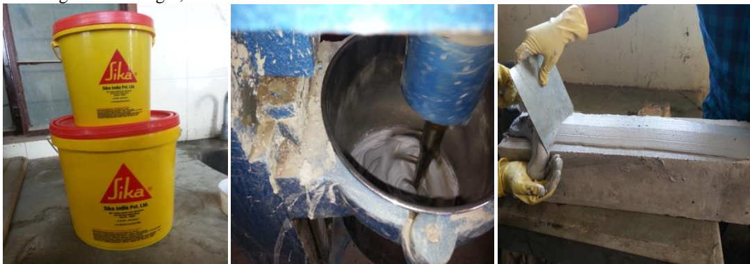
Fig. 5: Epoxy materials applied on beam
